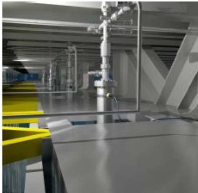
Figure 13—Illustration of sensors mounted on conductor of the well
